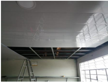
Maintenance and change of the ceiling to PVC.
