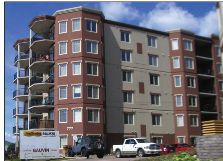
Typical Moncton housing renting for $1,150 per month
